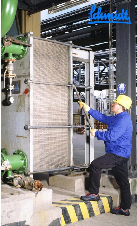
SIGMA plate heat exchanger
